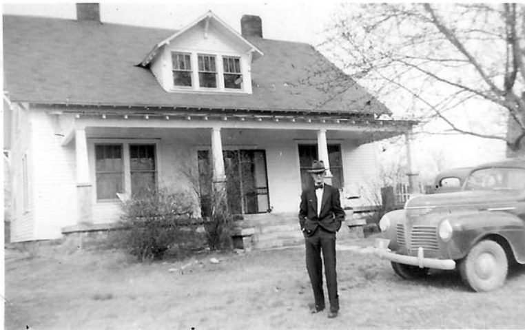
Granddaddy Hardison in front of the house several years after the fire. The fire was under the roof on the back of the house.
